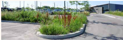
Bioswales capture and naturally filter rainwater
