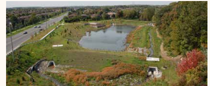
Stormwater management with quality and quantity controls at Pioneer Pond
