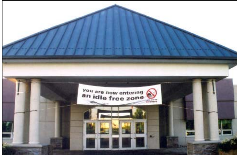
Figure 3: Idle-Free banner displayed over main entrance of the Town of Newmarket's municipal building.
