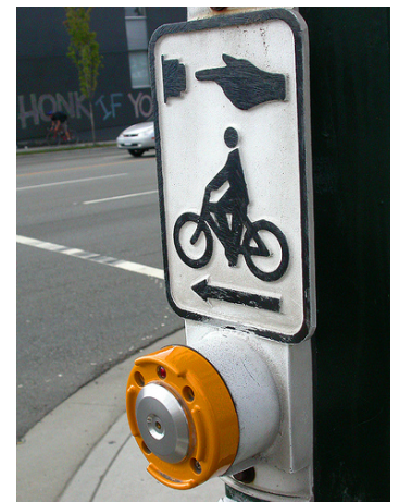
A CYCLIST PUSH BUTTON ALLOWS BICYCLISTS TO ACTIVATE TRAFFIC SIG- NALS WITHOUT DIS- MOUNTING THEIR BICY- CLE.
