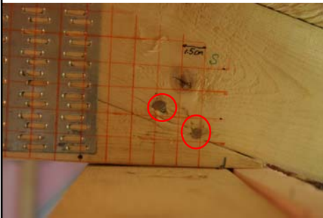
A typical toe-nail roof to wall connection in the test house
